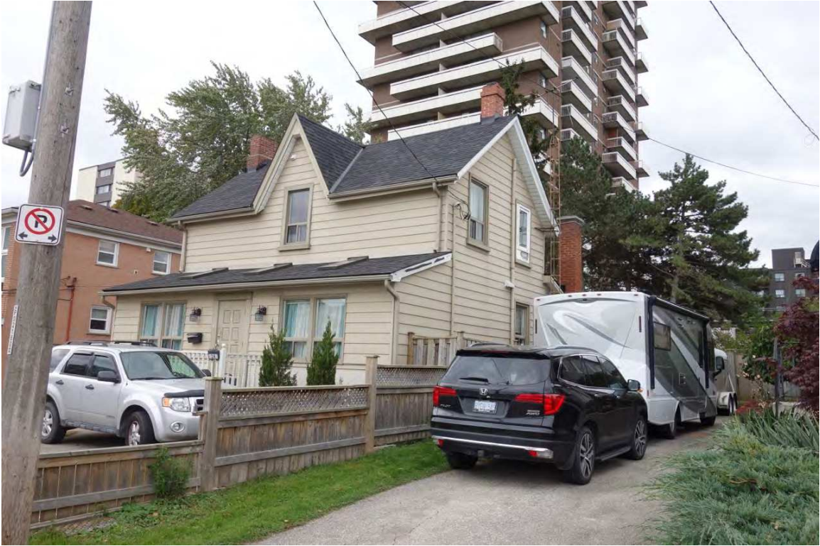
Figure 11: 24 Ann Street - EXTERIOR – front and north side elevation
