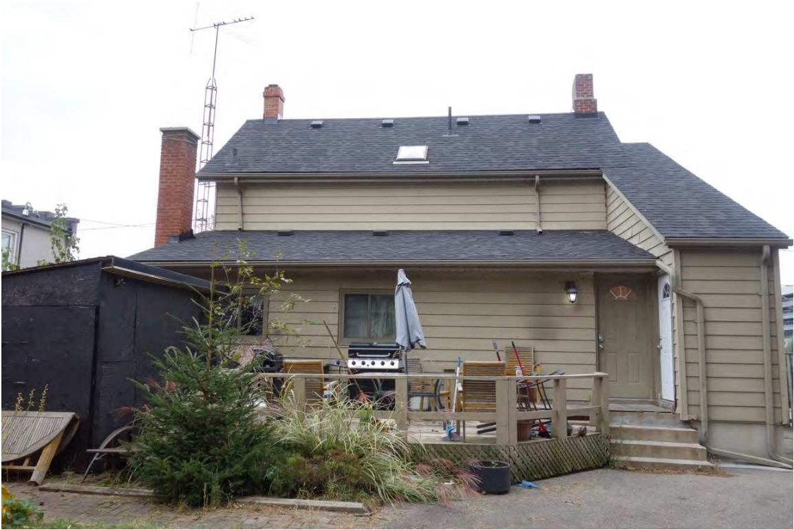
Figure 13: 24 Ann Street - EXTERIOR – rear elevation
