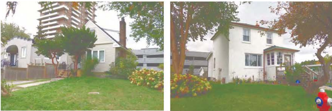
Figure 5: 24 Ann Street – CONTEXT – adjacent residential properties to the north
