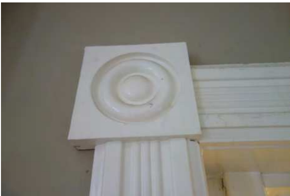
Figure 36: 24 Ann Street - INTERIOR - 2 nd FLOOR - living room - wood door trim
