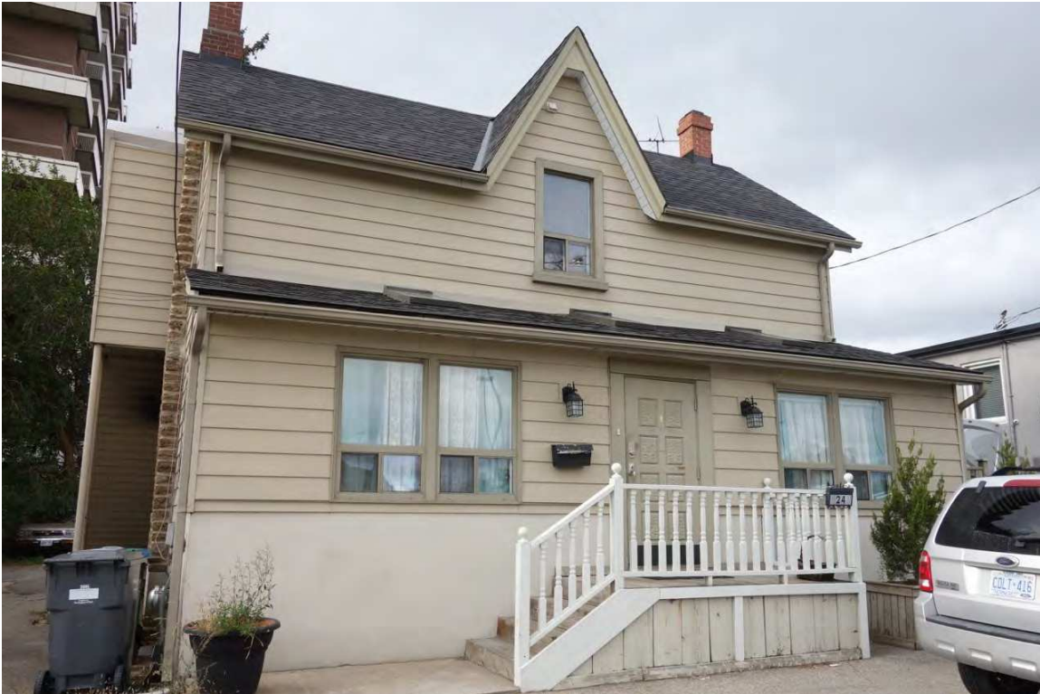
Figure 7: 24 Ann Street - EXTERIOR – main elevation facing Ann Street
