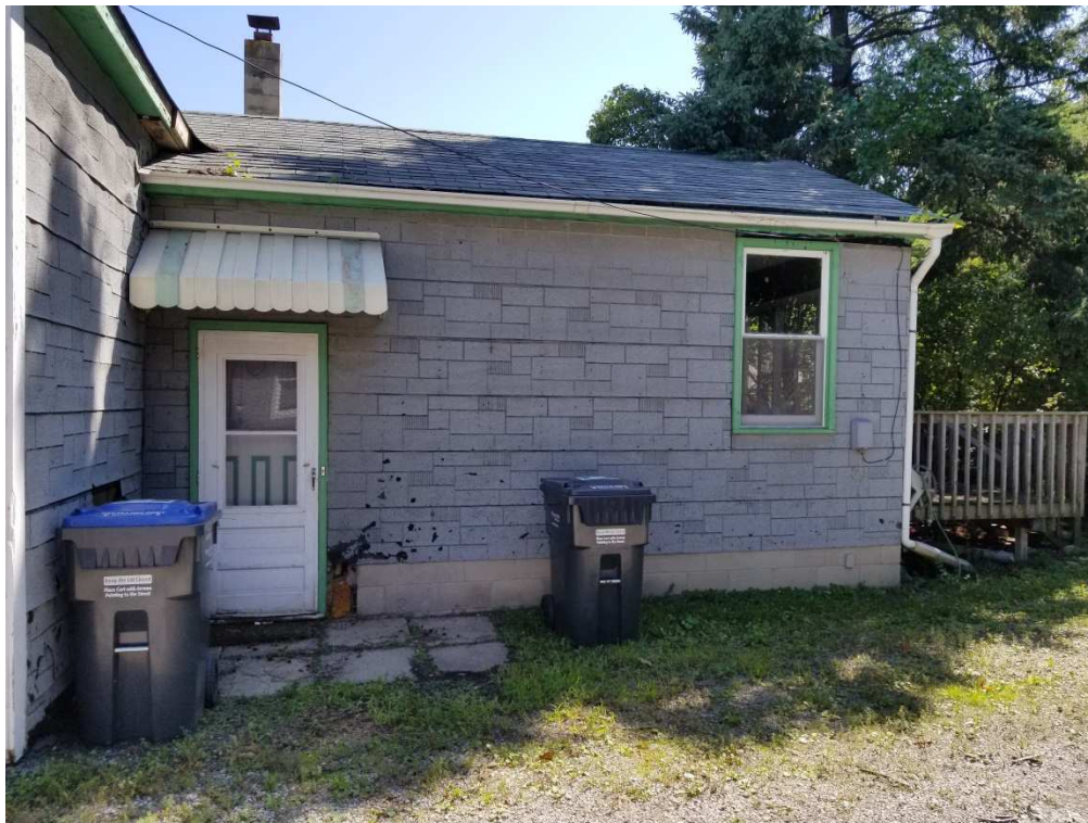
PARTIAL NORTH ELEVATION
