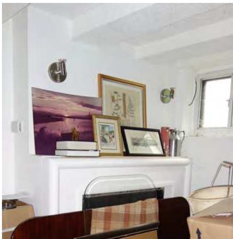
Figure 41: 24 Ann Street - INTERIOR – BASEMENT – exposed beams with modern spray stucco finish – modern fireplace and windows
