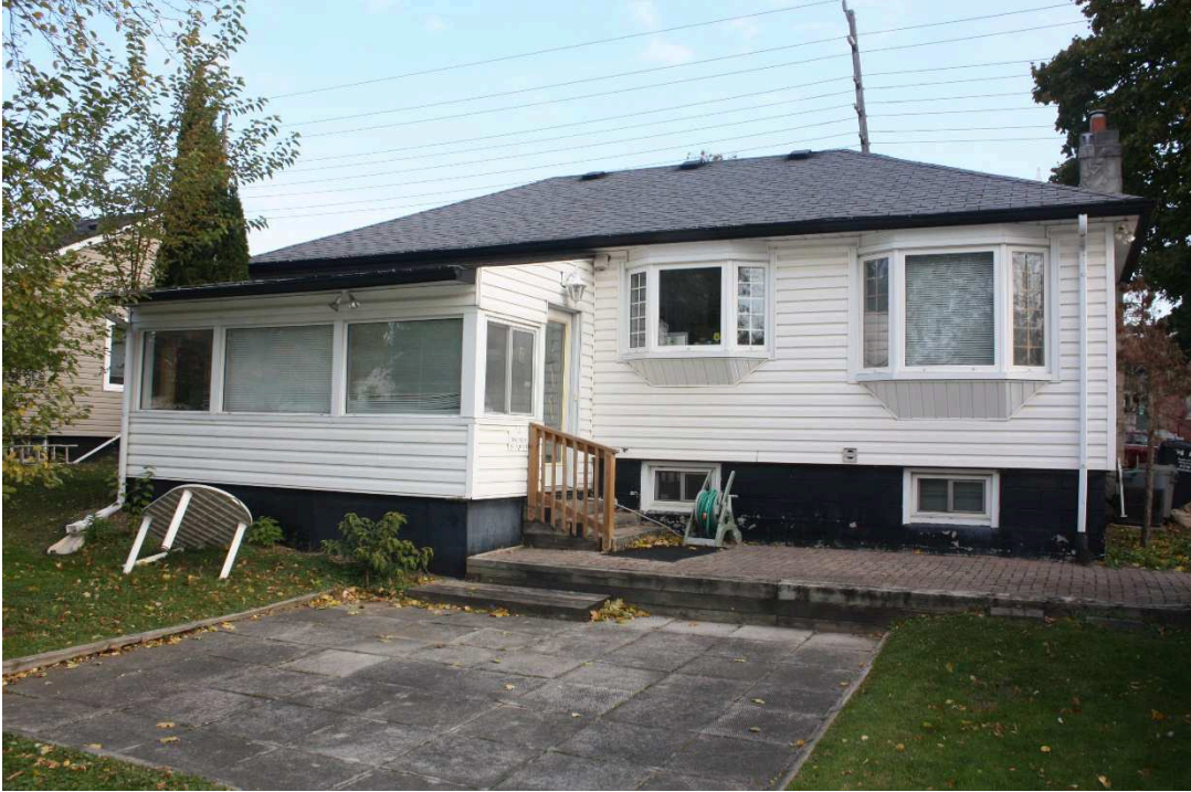
Figure 18 The rear or west façade of 70 Queen Street South. (Photo by author, October 2018.)
