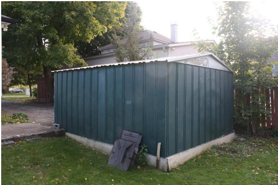
Figure 28 The north side and rear of the utility shed at 70 Queen Street South. (Photo by author, October 2018,)
