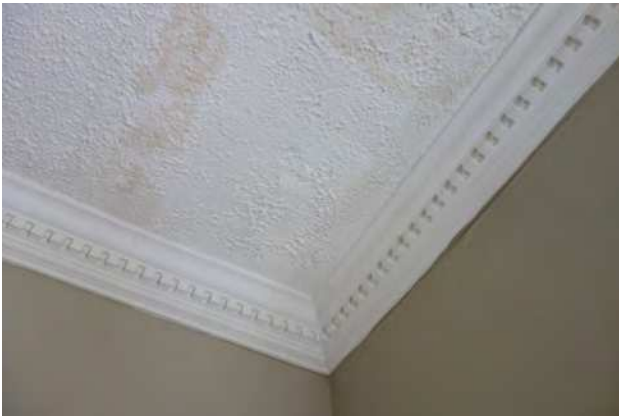
Figure 37: 24 Ann Street - INTERIOR - 2 nd FLOOR - bedroom - wood window trim & PVC crown moulding
