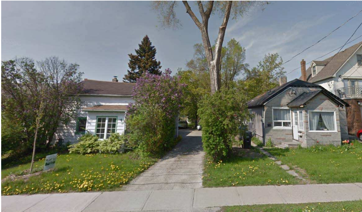
STREETSCAPE - 32 AND 34 QUEEN ST. S.
