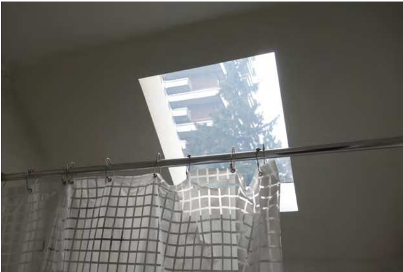
Figure 38: 24 Ann Street - INTERIOR - 2 nd FLOOR - bathroom - modern skylight
