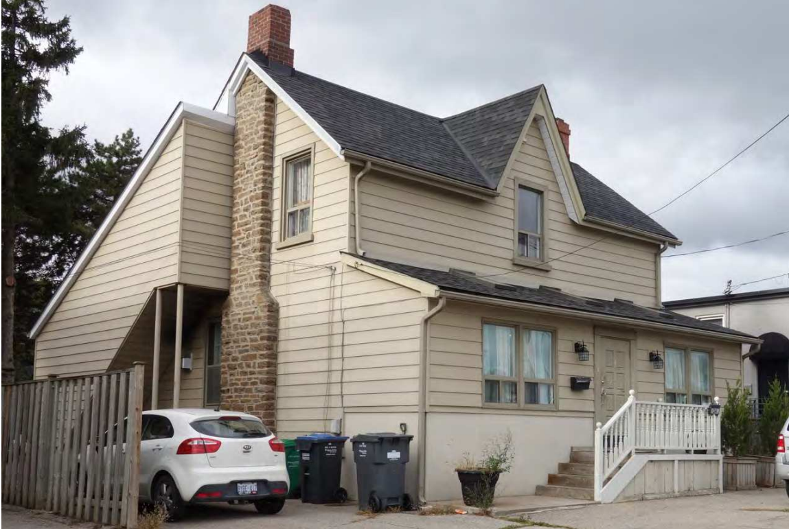
Figure 9: 24 Ann Street - EXTERIOR – front and south side elevation – external staircase on south elevation
