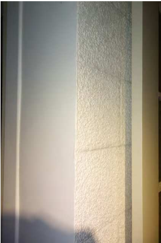
Figure 40: 24 Ann Street – BASMENT – concrete block walls
