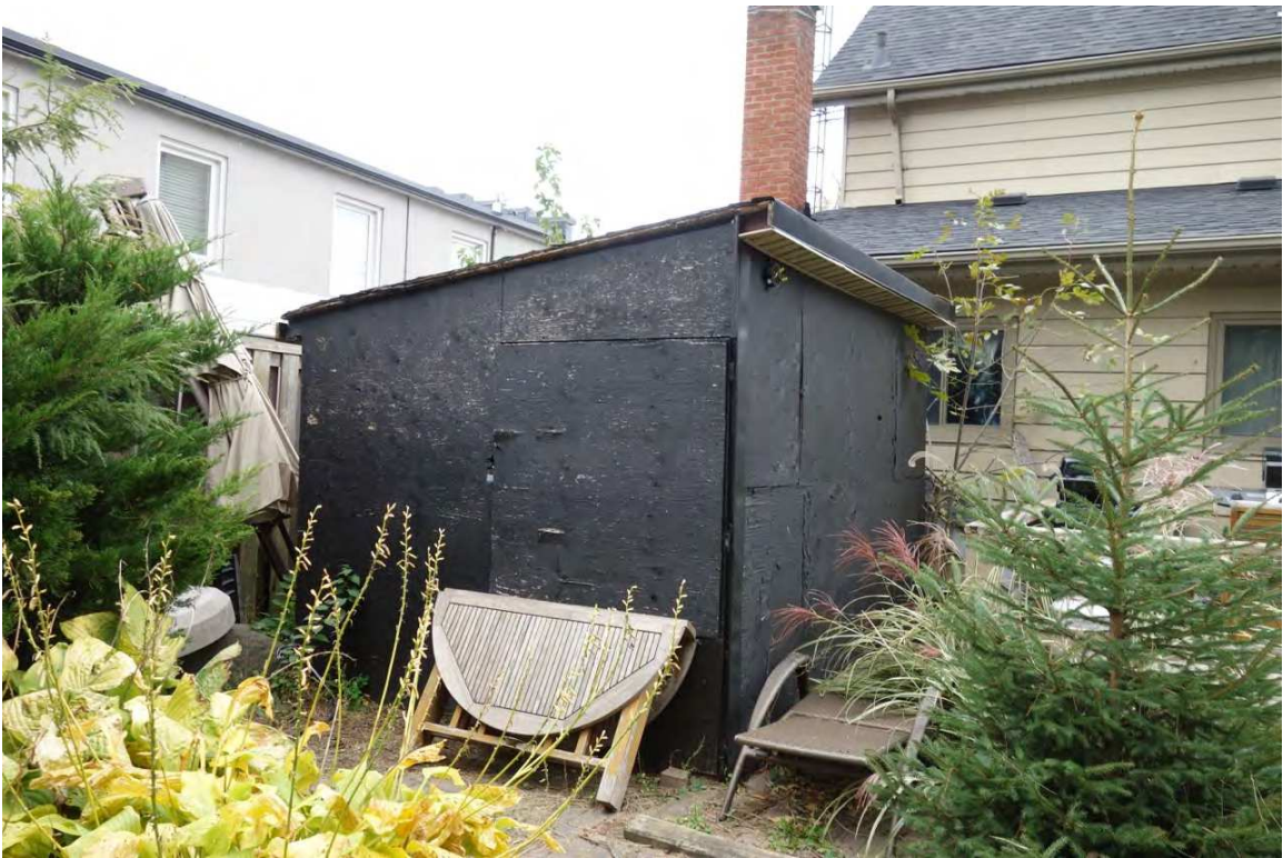
Figure 14: 24 Ann Street - EXTERIOR – plywood-clad shed in the rear yard
