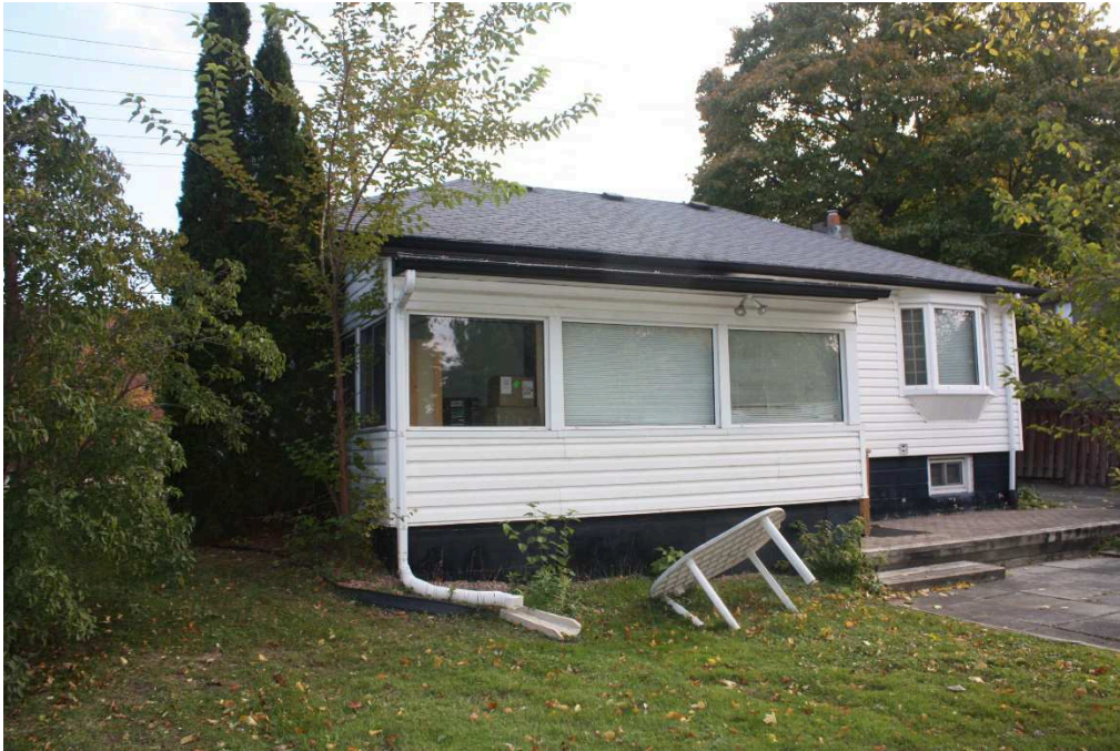
Figure 32 The juniper tree on the north façade of 70 Queen Street South. (Photo by author, October 2018.)
