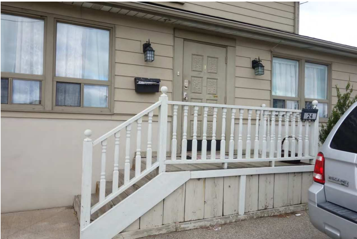
Figure 8: 24 Ann Street - EXTERIOR – stairs to front entrance
