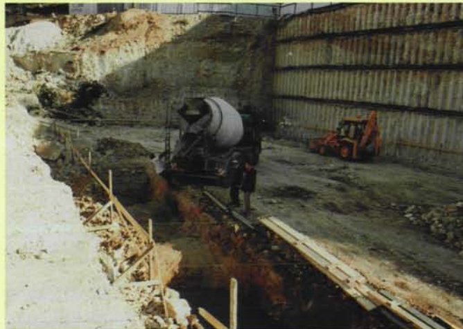
The laying of the foundations of the new Yad Vashem Archives
