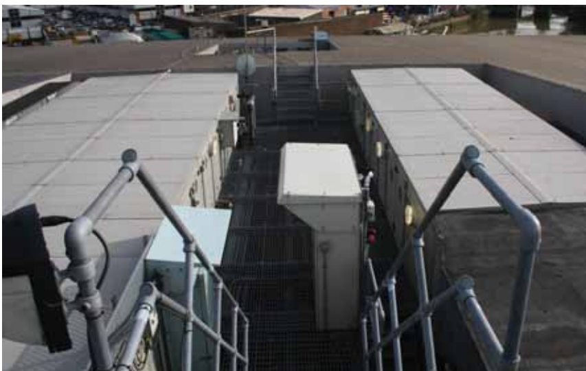
RIGHT: The ahus are squeezed into a pit on the building's roof. ABOVE LEFT: A baffle was added to prevent air short circuiting between the unit's intake and exhaust louvres. ABOVE RIGHT: Since completion a curved scoop has been added to throw the exhaust air clear of the roof pit
