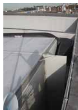
RIGHT: The ahus are squeezed into a pit on the building's roof. ABOVE LEFT: A baffle was added to prevent air short circuiting between the unit's intake and exhaust louvres. ABOVE RIGHT: Since completion a curved scoop has been added to throw the exhaust air clear of the roof pit
