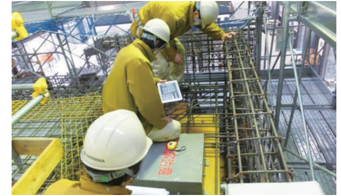
3 Practical training using RC mock-up
