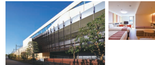
Hotel Dream Gate Maihama Annex
