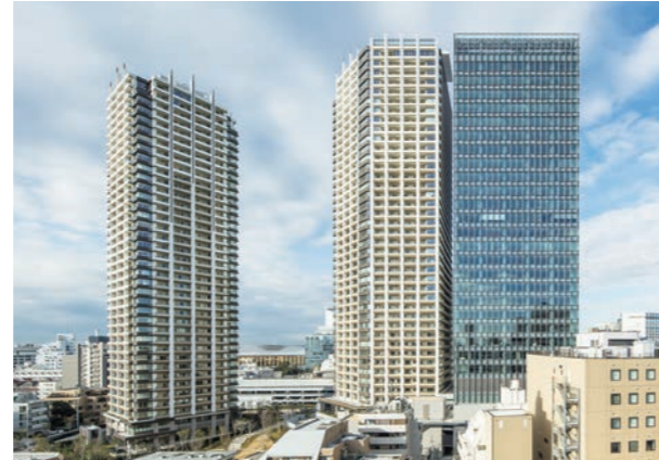
Basic design: Nihon Sekkei Construction design: Takenaka Corporation
