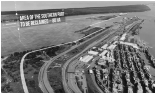
b) preliminary layouts of the reclaimed territories in the southern part of Klaipeda port
