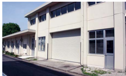
▶共同教育研究棟▶ Joint Education and Research Center
