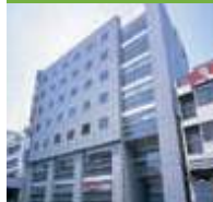
Matsudo City Bldg.
