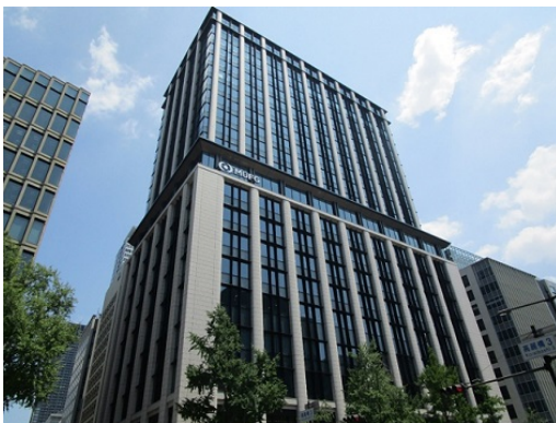
Exterior of the Osaka Building
