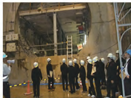
建設工事現場の見学 Visit to a Construction Site
