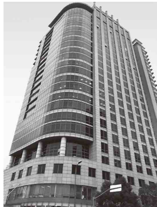
KCHが入る上海Long Feng Building
