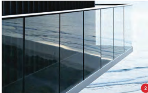
GLASS RAILING - DARK BRONZE @ WEST & SOUTH DECKS
