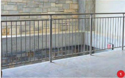
SITE RAILING @ SITE RETAINING WALL
