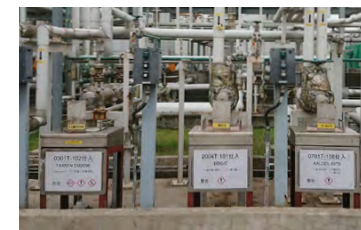
GHS labeling at raw materials intake ports (example)
