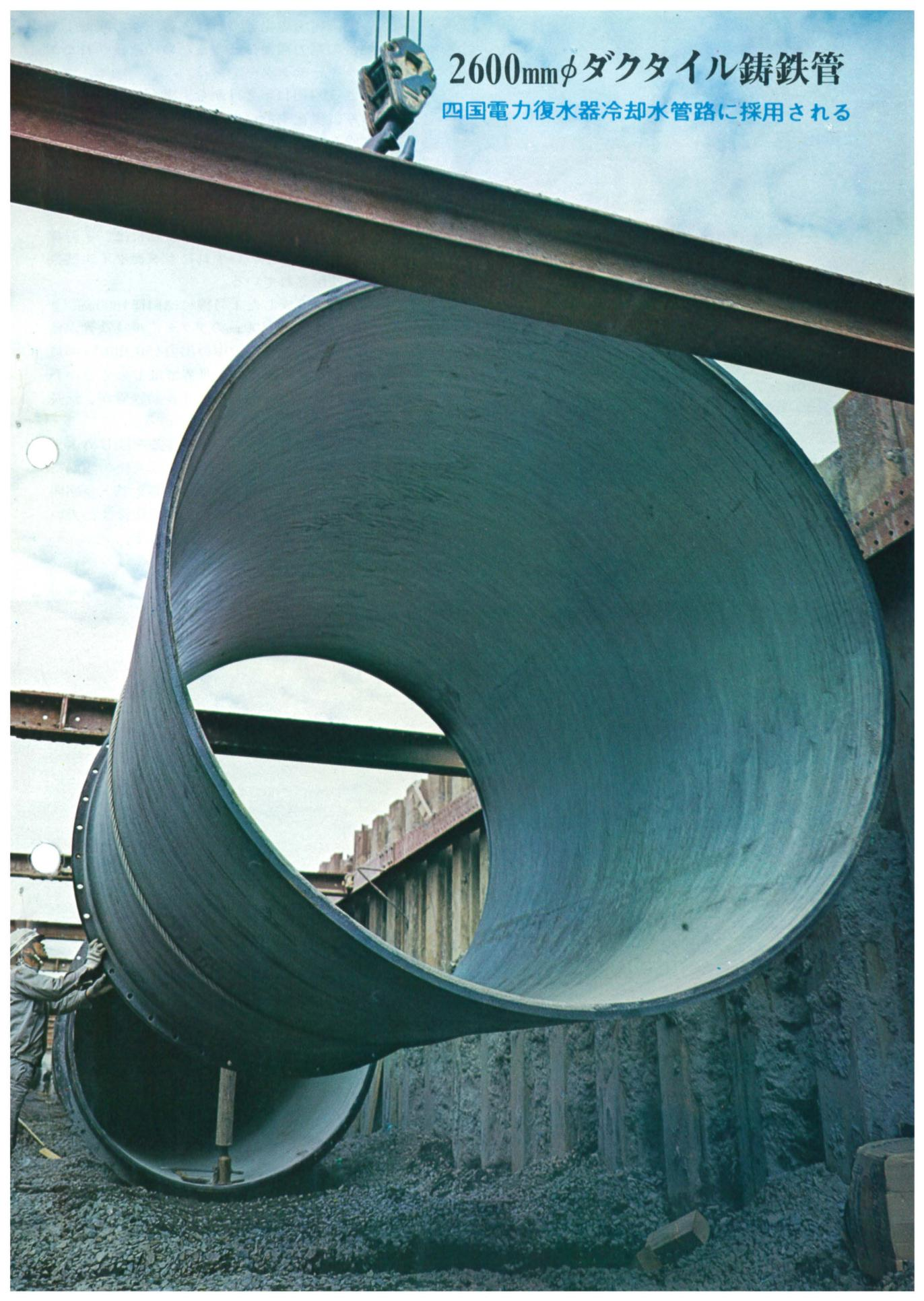
A large, dark-colored ductile cast iron pipe is being lifted by a crane hook. The pipe is curved, showing its massive scale. In the background, there are steel beams and a worker in a white protective suit. The ground is covered with gravel.
