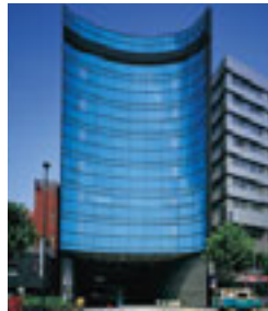
I-33 IKEBUKURO YS BUILDING 池袋YSビル
