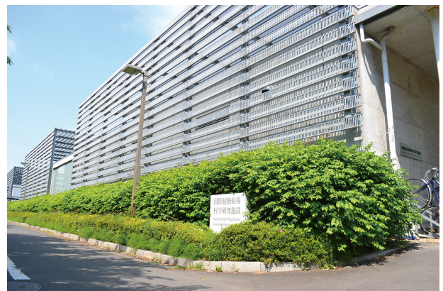
Fig. 1. Building view of the International MegaGauss Science Laboratory (C-building) at ISSP.
