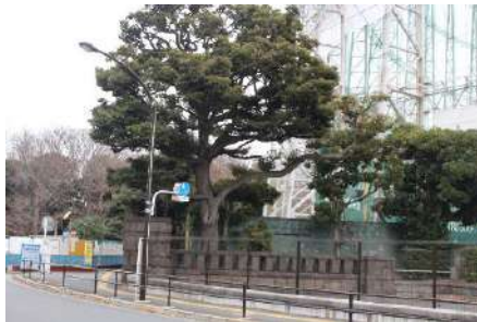
Photo 29 Kasumigaoka gate (April 2023)
