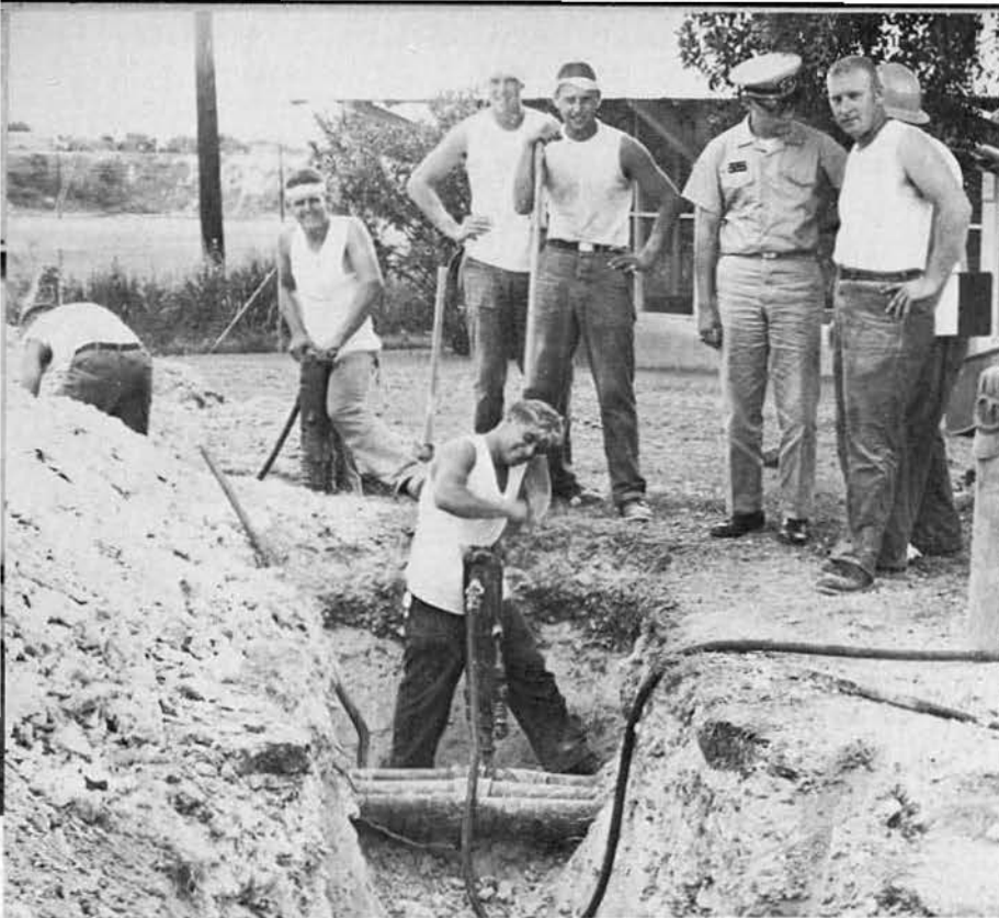
Villamar Pipe Line
