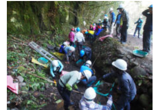
Removal of sediment from waterways in Yase, Mifunemachi, Kumamoto in 2016' earthquake.
