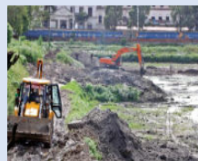
Use of bulldozer and excavator
