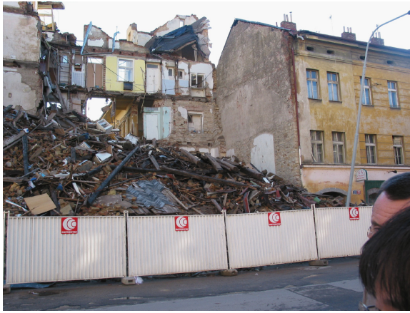
Photo 1 Building damaged by flood inundation
