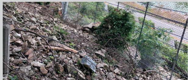
設計した崩壊土砂防止柵により土砂災害を防いだ事例（道路防災点検・防災設計） Example of sediment disaster protection by designed collapse prevention fence (Inspection and design for road disaster prevention)
