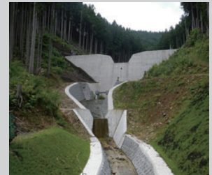
不透過型堰堤 Impermeable type SABO dam
