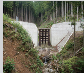
透過型堰堤 Slit type SABO dam
