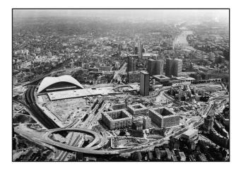
Fig. 2: 1971 aerial photograph shows the agony of construction endured by the pioneering residents and office workers. Note the even height and floor plates of the towers. The *dalle* is taking shape in front of the CNIT building, the freeways and suburban railroad are already complete. (EPAD photo courtesy De Facto)
