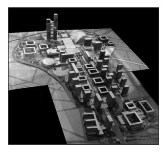
Fig. 1: The 1964 Master Plan model from the east, showing the theme tower and CNIT at the back. Note the uniform dimensions of the residential squares and the office towers, and their symmetrical arrangement along the *dalle*, or pedestrian mall.
