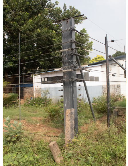
Fig: A steel-rope fence
