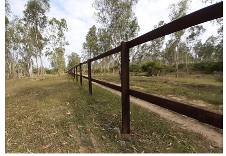
Fig: A rail-track fence.
