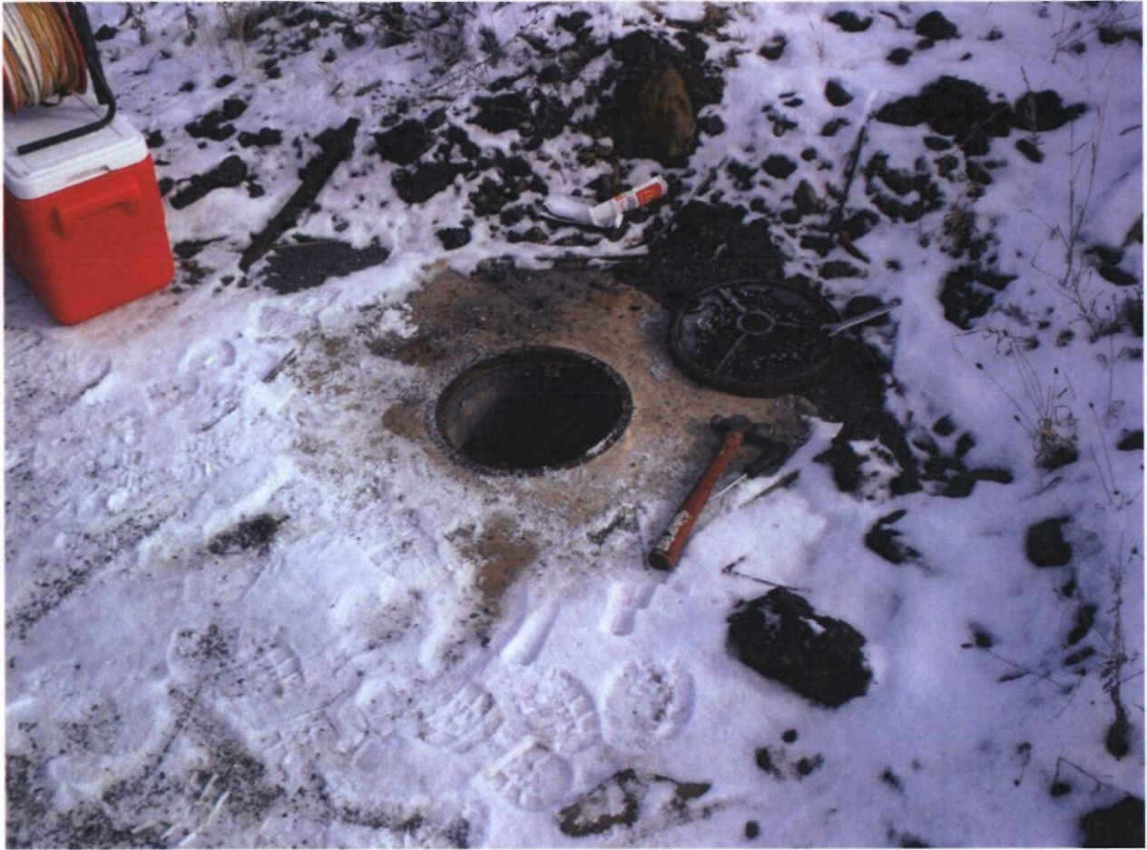
Borehole 11, near HWAS Service Station. Located along Route 315.
