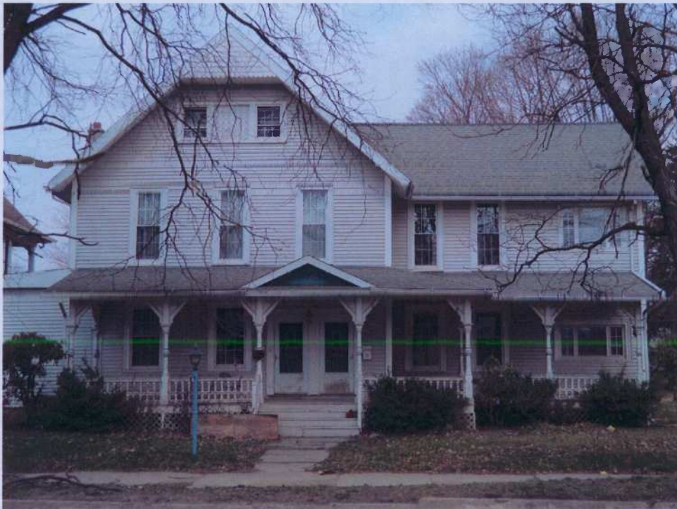
Photo 10- 216 Wyoming Avenue, looking north
