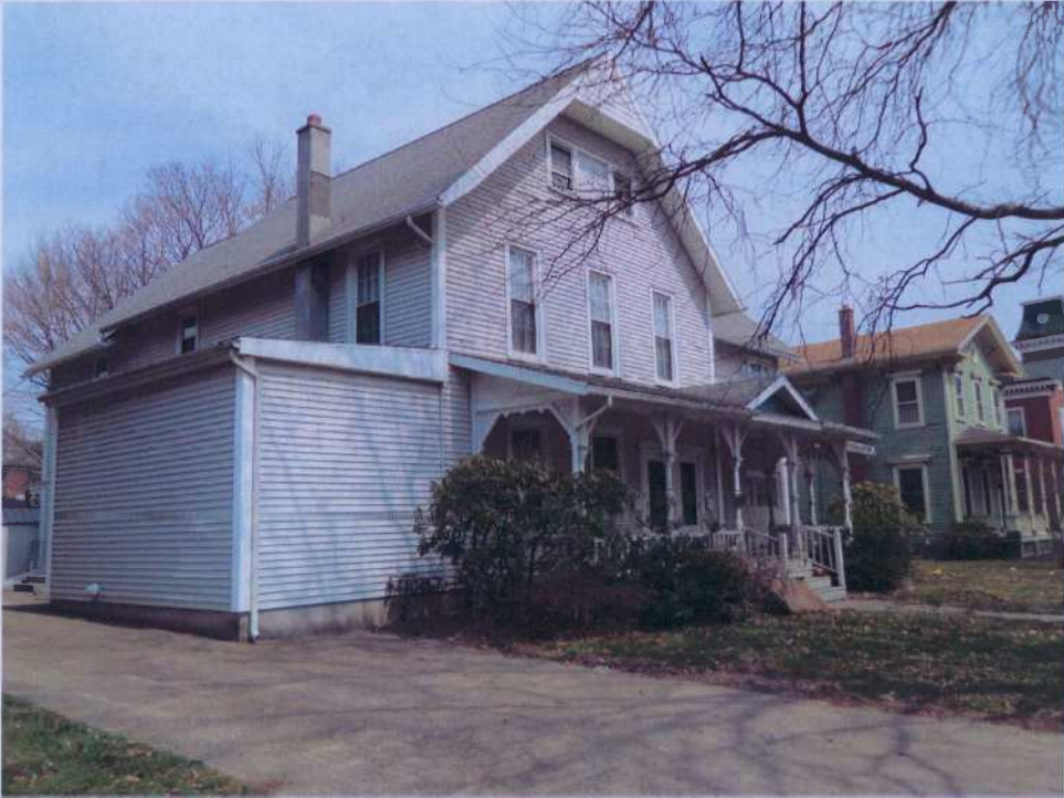
Photo 11- 216 Wyoming Avenue, looking northeast
