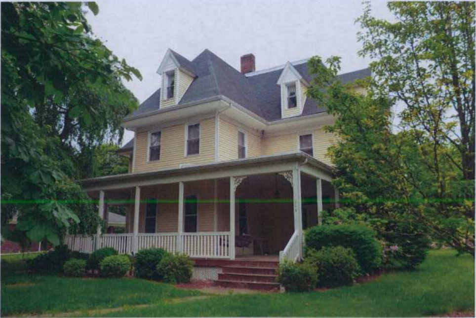
Photo 8- 804 Susquehanna Avenue, looking southwest
