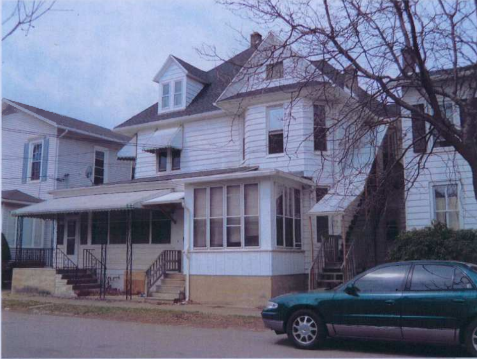
Photo 17- 320-322 Race Street, looking west
