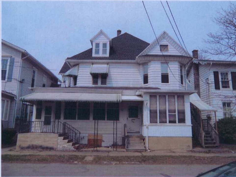
Photo 15- 320-322 Race Street, looking southwest
