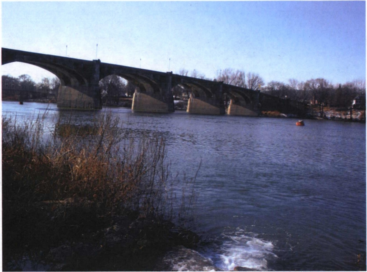
View of Susquehanna River where Butler Mine Tunnel outfall discharges to river.
