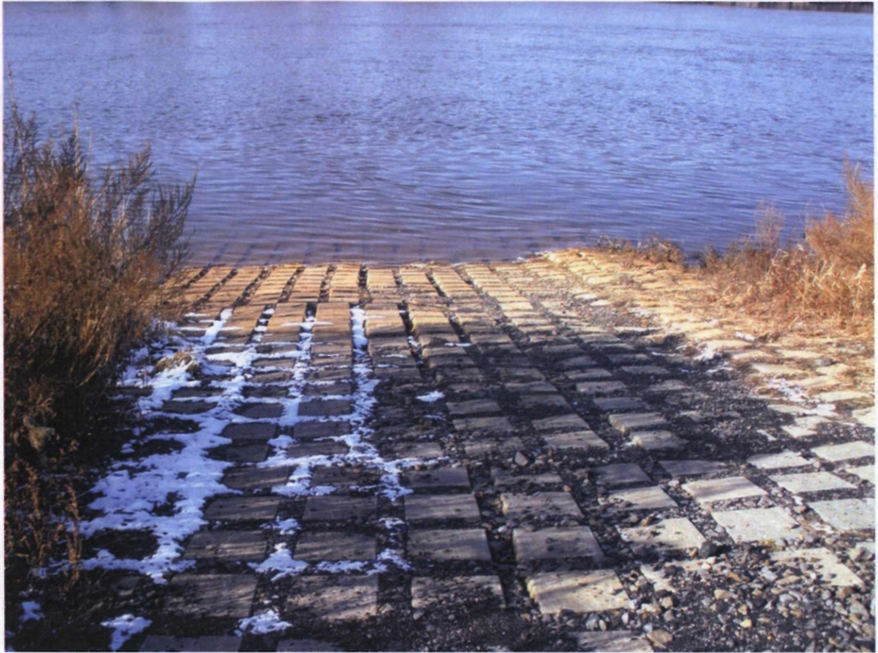
View of boat ramp to Susquehanna River; one of a number of features constructed on the river bank to facilitate potential future oil responses.
