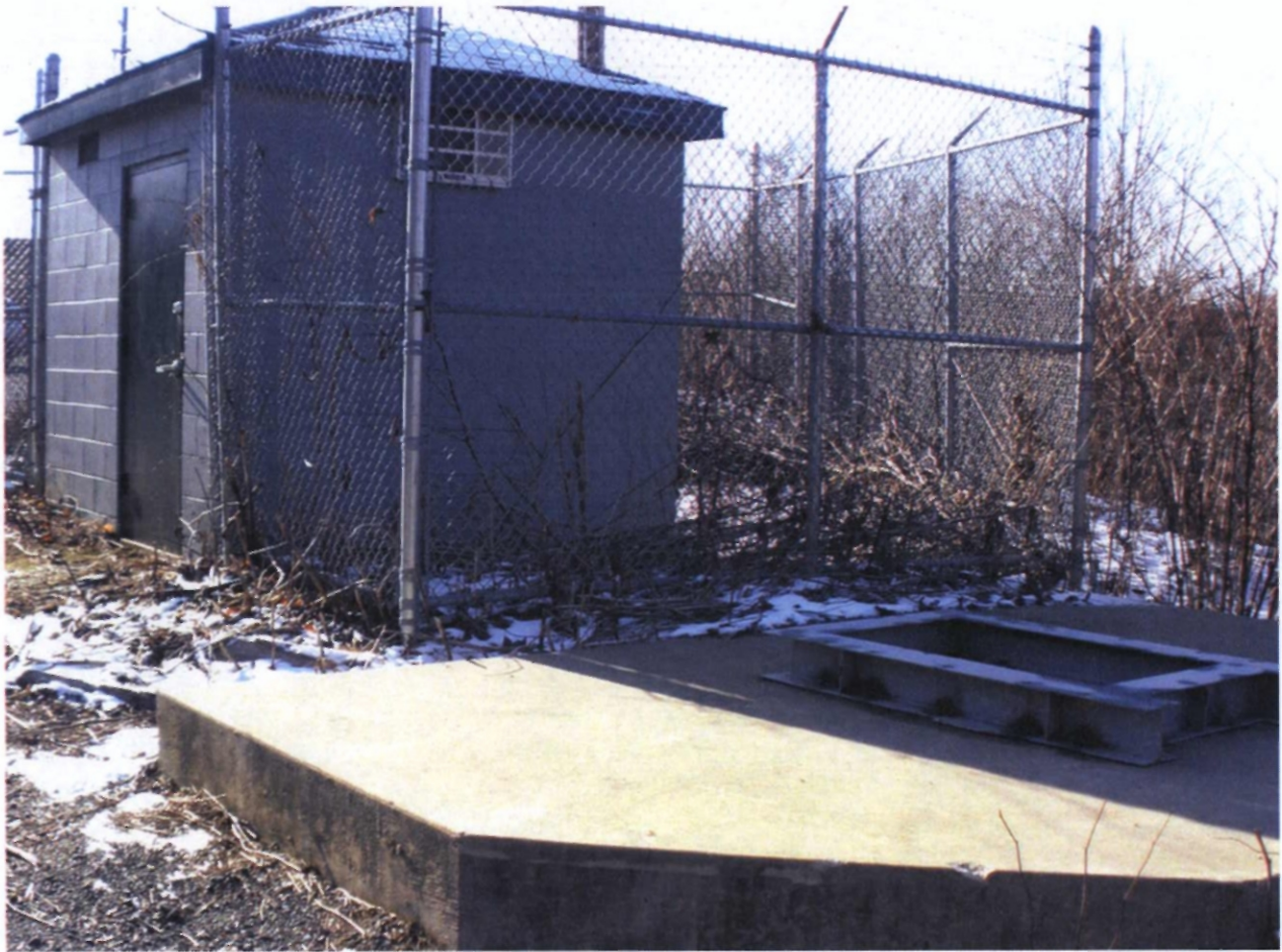
View of monitoring building, located approximately above the Butler Mine Tunnel near where the Tunnel discharges into the Susquehanna River. In foreground is a concrete pad mounted winch pad, used to control lines during training activities and potential on-river oil responses.
