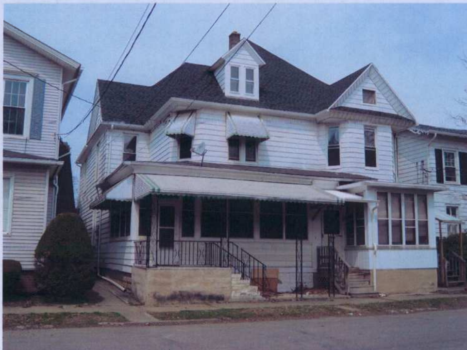
Photo 16- 320-322 Race Street, looking northeast
