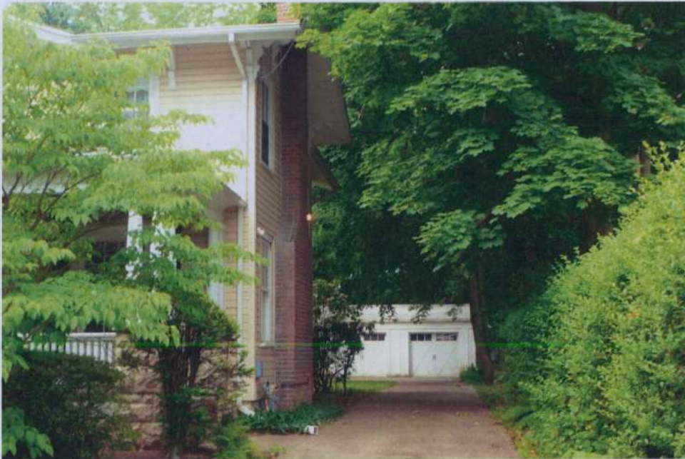
Photo 4- 21 Exeter Avenue, looking southwest
