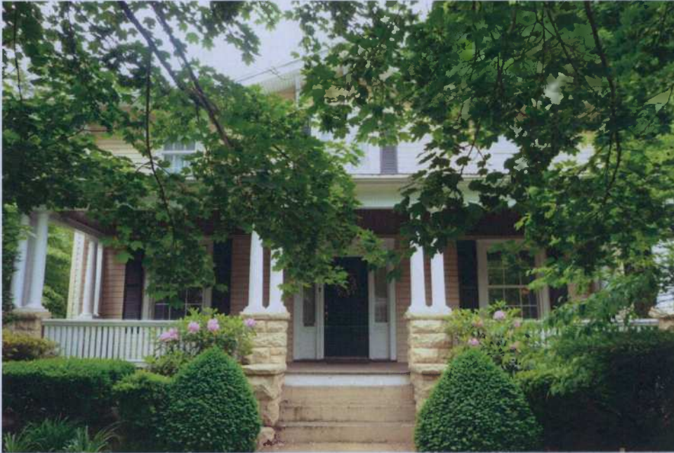
Photo 5- 21 Exeter Avenue, looking southwest
