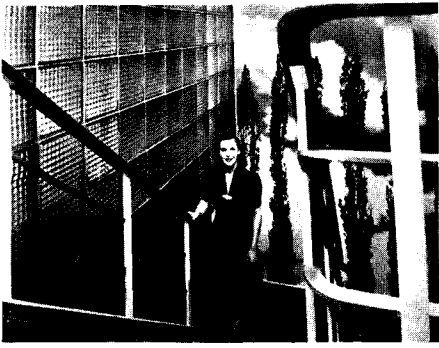
The fluorescent tube is several times more efficient than the incandescent filament. Here it is built into a two-story glass-block wall.
