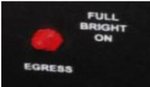
Figure 6.8. Emergency Egress Controls.
