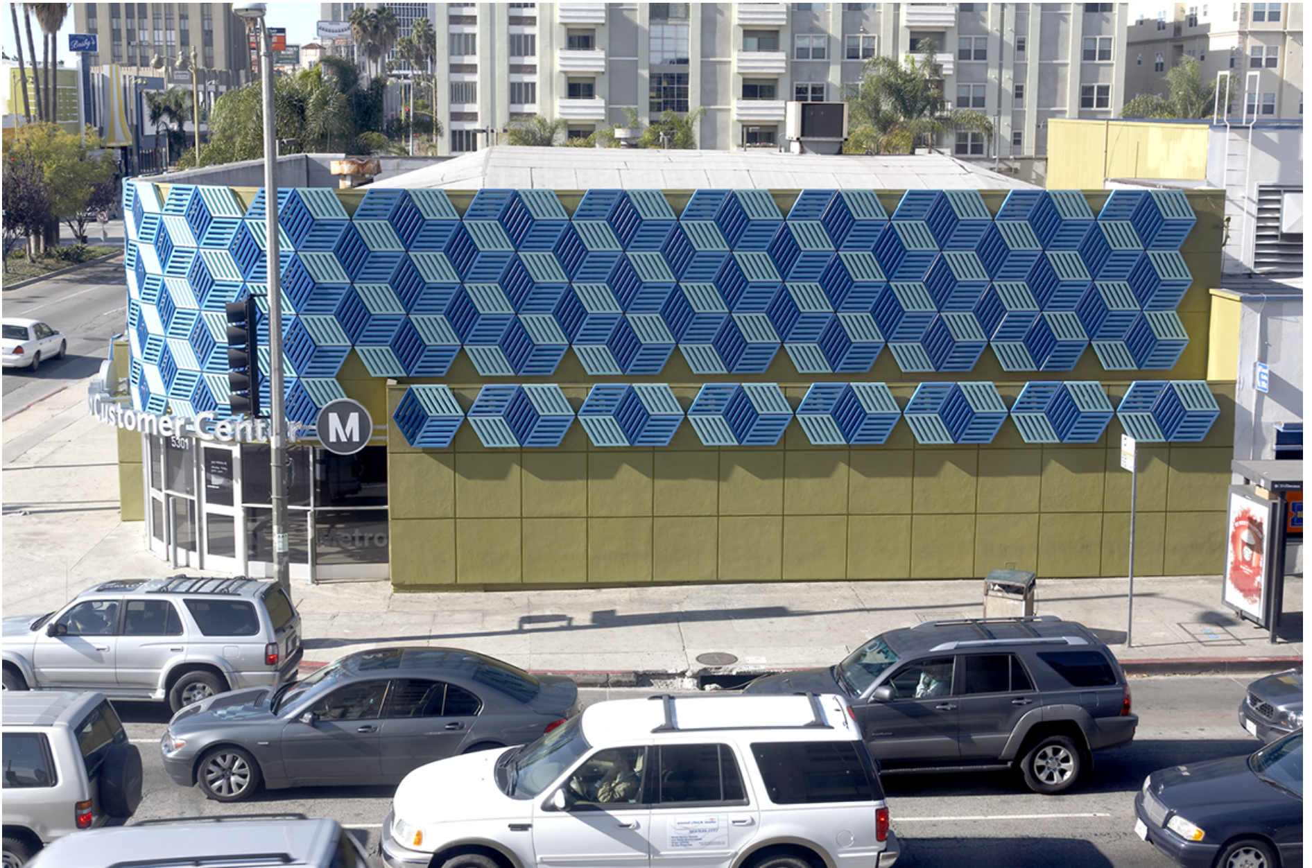
Attachment C: Wilshire Customer Center Artwork Panels and Signage Installed 01.18.13
