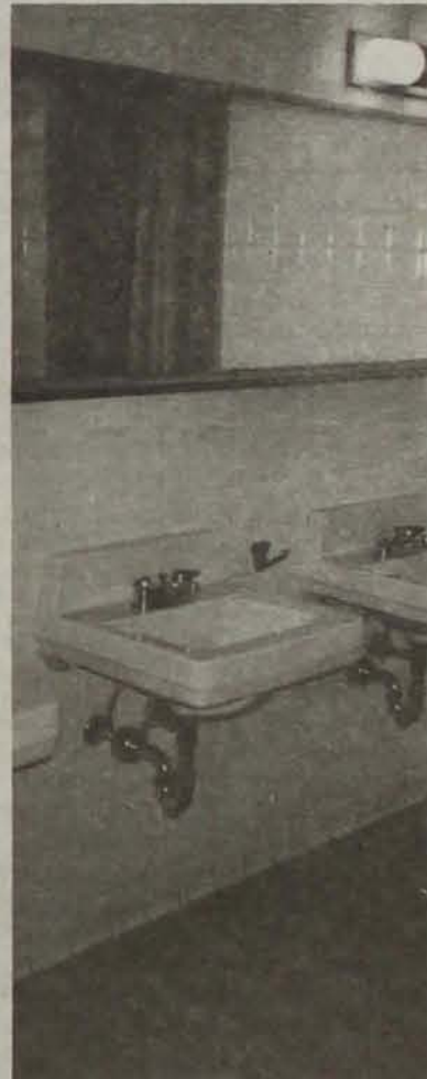
Wash basins and mirror in bathroom at each end of the floor. Each will be designated for men and women.
