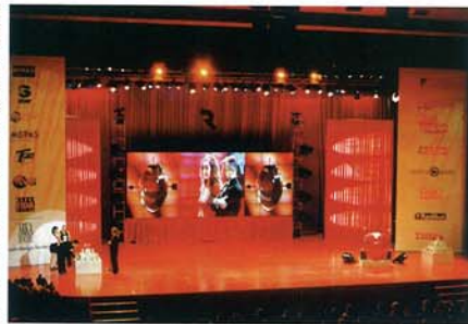
An impressive 5 x 10 videowall installed by Electrosonic's distributor in Turkey, Visions Communication Ltd. It (and two other 3 x 3 walls not in this picture) supported the Crystal Apple Advertisement Festival. The cubes were Sony RVP411, and the processing Electrosonic PICBLOC-3.
