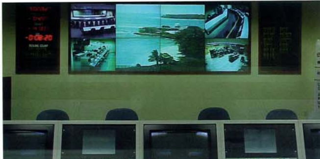
Eight ProDigital 40 inch projection units with built-in image scaling make up the main display in the conference area of the Mission Control Room on Meck Island. The display is typically used to show a mixture of 1280x1024 computer workstation and video surveillance images, but this particular photo shows only video images.
