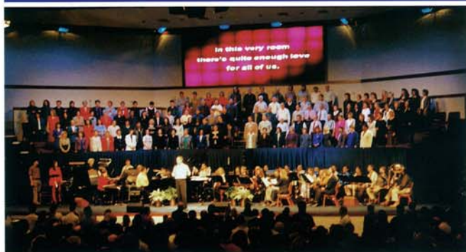
The People's Church in Franklin TN use a 4x8 Electrosonic videowall installed by Allied Sound Inc. It shows hymn lyrics, paging information and both live and recorded video. IMAGEMASTER™ processing is used.
