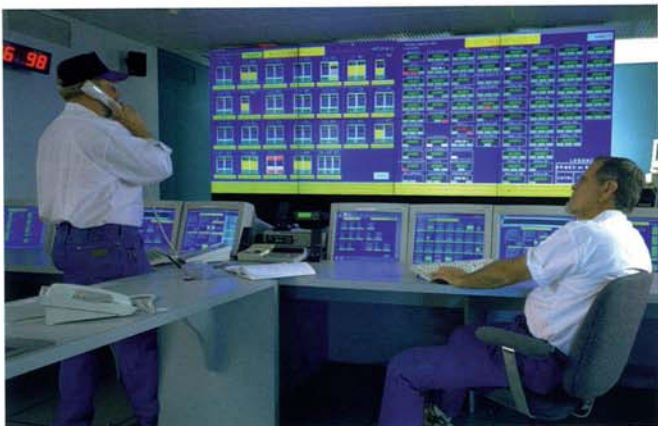
The display at LVVWD uses eight ProDigital™ 50 inch projection units with VECTOR™ processing, to give a 14ft wide display only 28 inches deep. Displayed resolution is 3200x1200, 32 different data and video sources can be displayed. The ProDigital displays use Texas Instruments DLP™ technology, to give a rock steady, evenly illuminated, and highly legible image.
