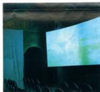
Metamorphosis at Vinopolis - a year in the life of a vineyard shown in just a few minutes on a 9m x 3m screen. Three Sony VPH-DSO projectors are used with electronic soft edge masking. The three synchronised video sequences run from Electrosonic server.
