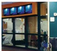
"Sea", one of four compact videowalls installed at Eggleston Children's hospital by Visioneering International.
