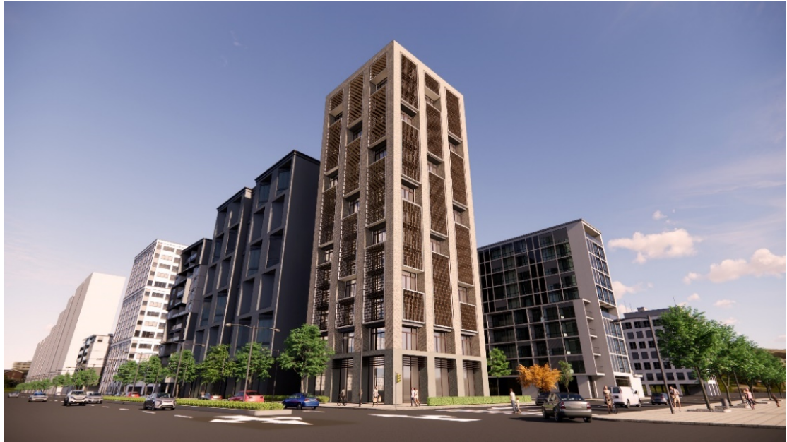
Figure 31. Apartment with dynamic shading screens at 7 am.
