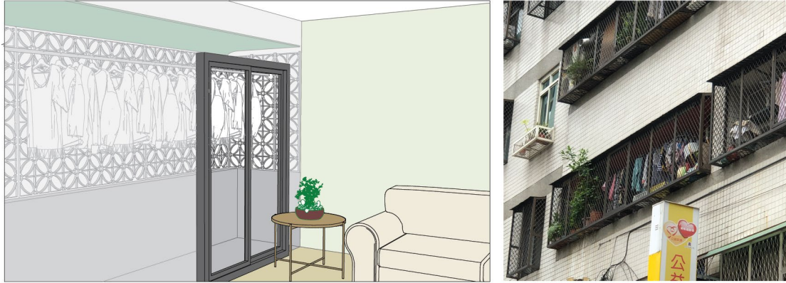
Figure 14. A utility space enclosed by a window grille.
