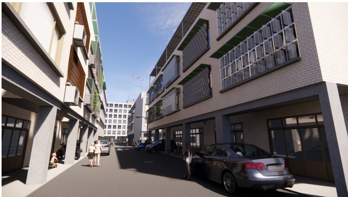
Figure 41. The townhouse with dynamic shading screens at 10 am.
