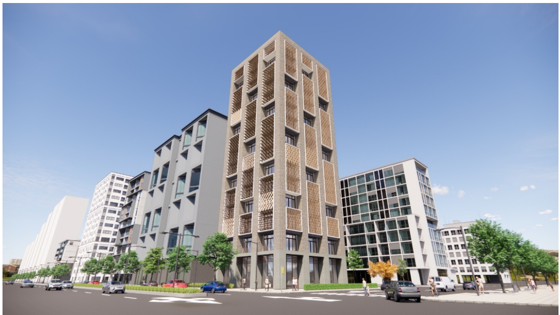
Figure 32. Apartment with dynamic shading screens at 10 am.
