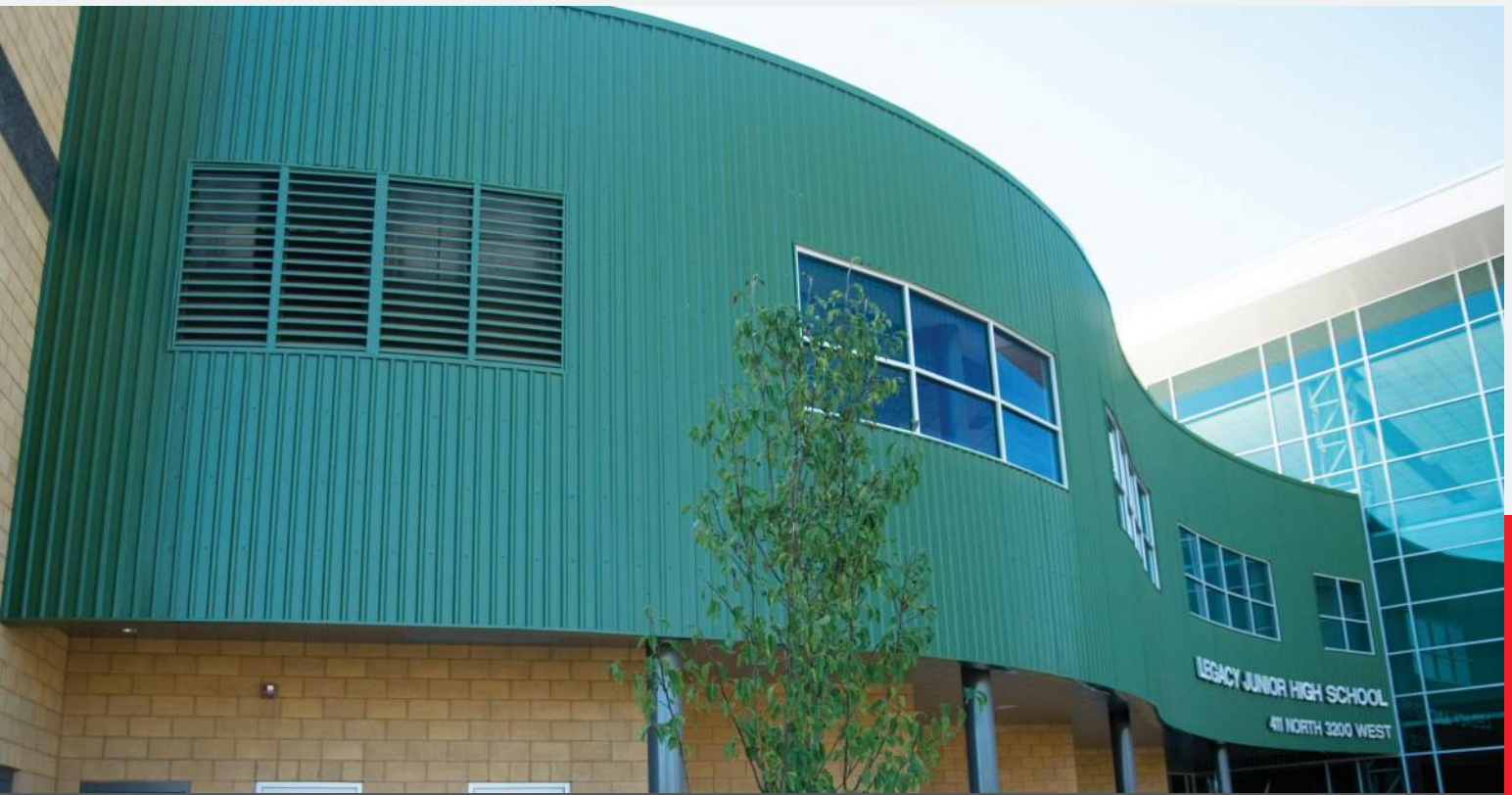
PROJECT: Legacy Junior High School LOCATION: Layton, UT PANEL PROFILE: PBU, Artisan® Series COLOR: Laurel Green, Tundra
