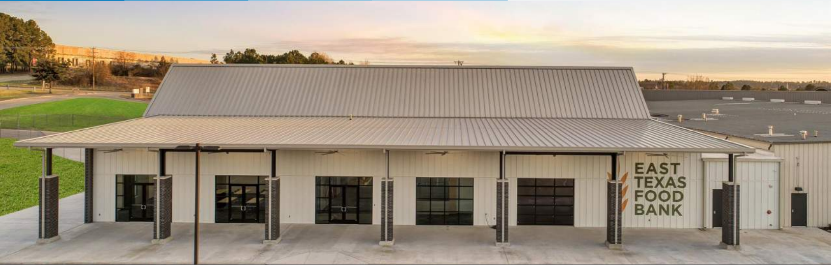
PROJECT: East Texas Food Bank LOCATION: Tyler, TX PANEL PROFILE: BattenLok® HS COLOR: Slate Gray
