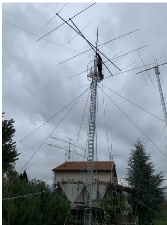
Aiming the 15m Yagi towards NA
