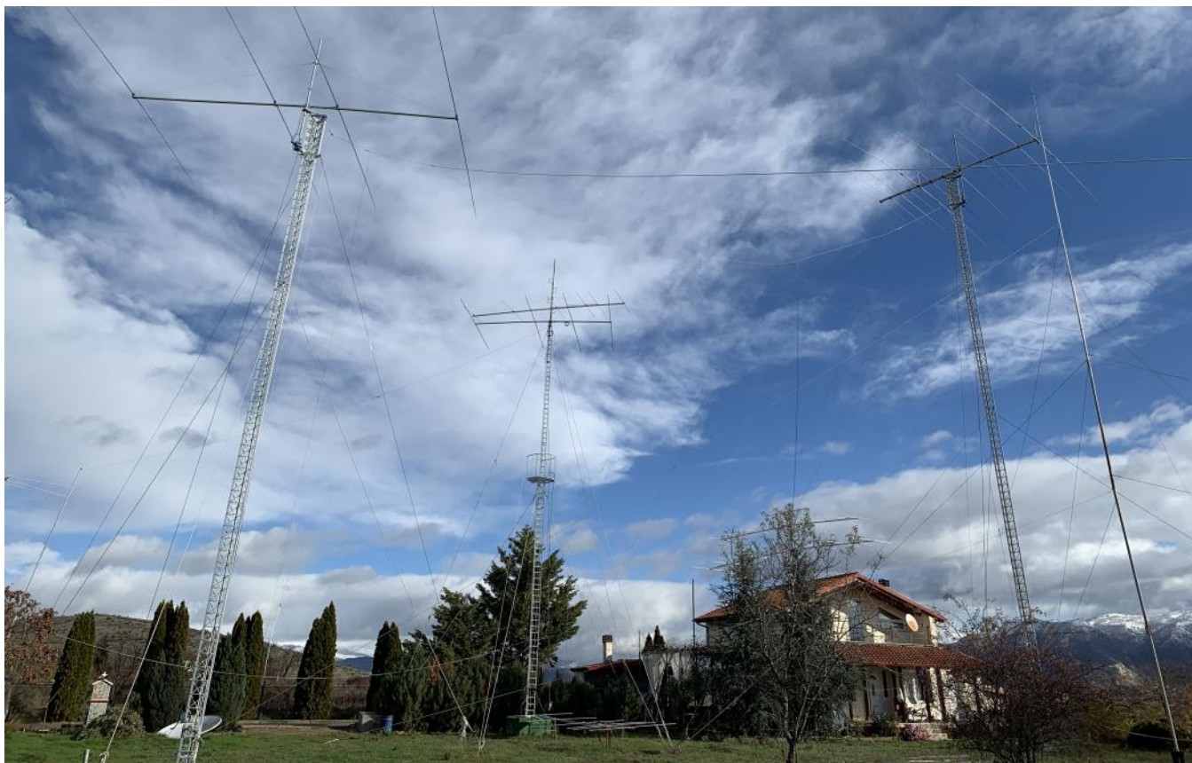
Some J42L antennas, 20 m tower, 15 m tower and Optibeam multibander tower. 40 m 4 el wirebeam is barely visible between 20 m tower and Optibeam tower.
