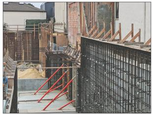
Supports and a retaining wall in the giant pit at Dolores and Fifth are not doing a good job supporting the adjacent, Carmel Foundation-owned apartments, according to the foundation's director
