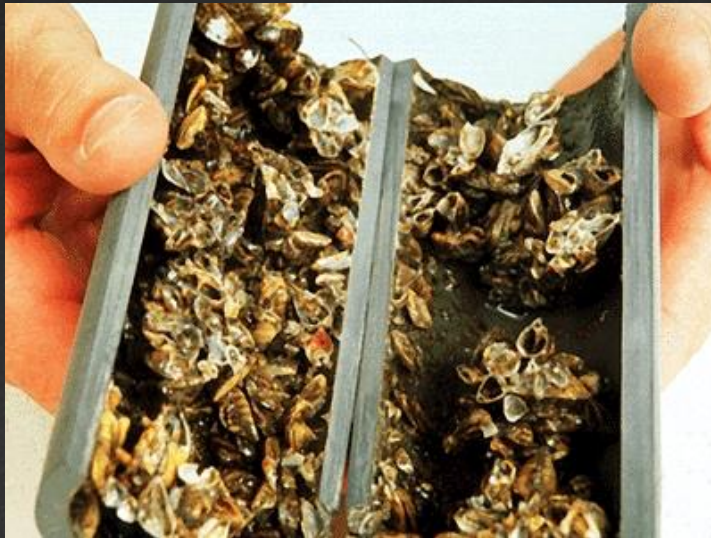
Dreissena in intake pipe
