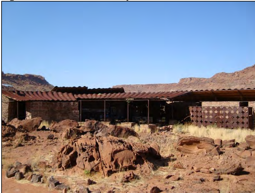
Figure 5: Visitor Centre at Twyfelfontein
