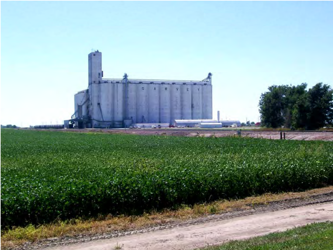
View of Garvey Elevator from Highway 6, looking southwest
