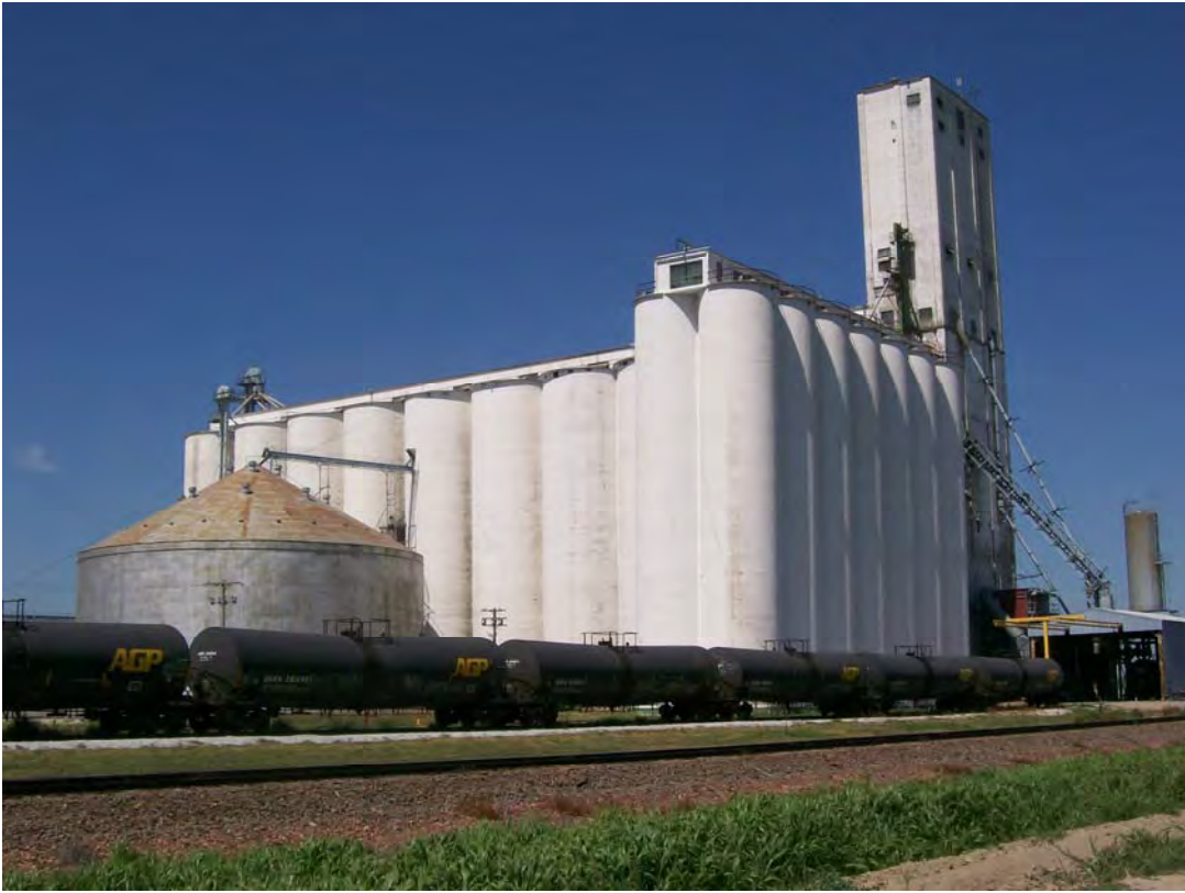
Garvey Elevator facility, looking northwest
