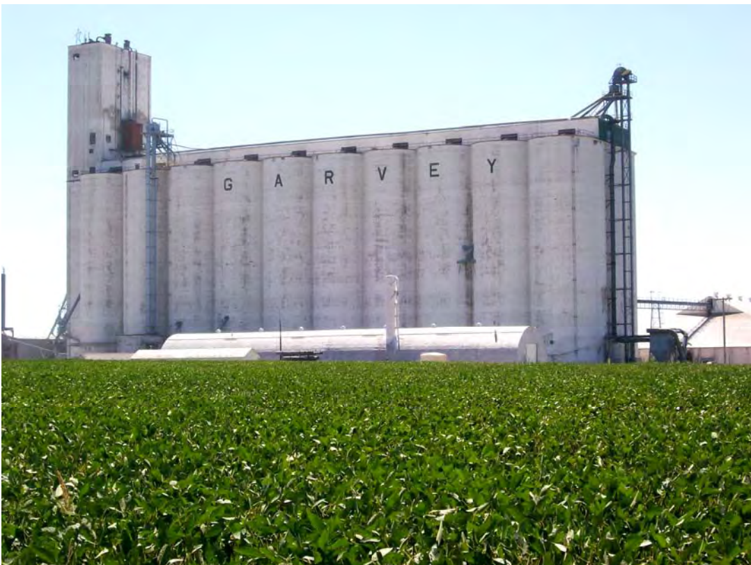
Looking south to the Garvey Elevator
