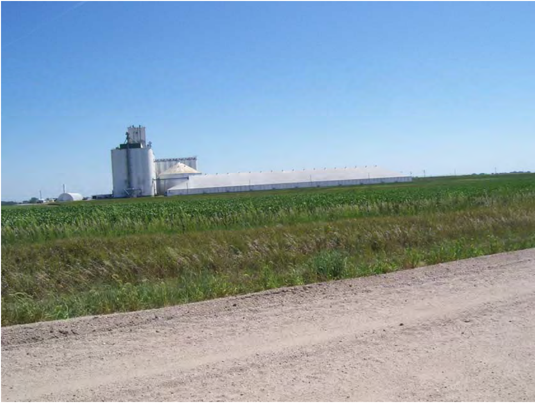
Distant view of Garvey Elevator facility, looking east from S. Marian Road
