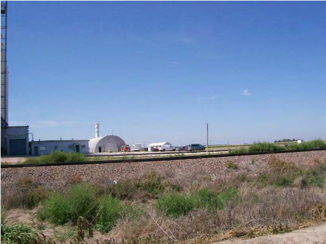
North portion of the Garvey Elevator facility, looking west
