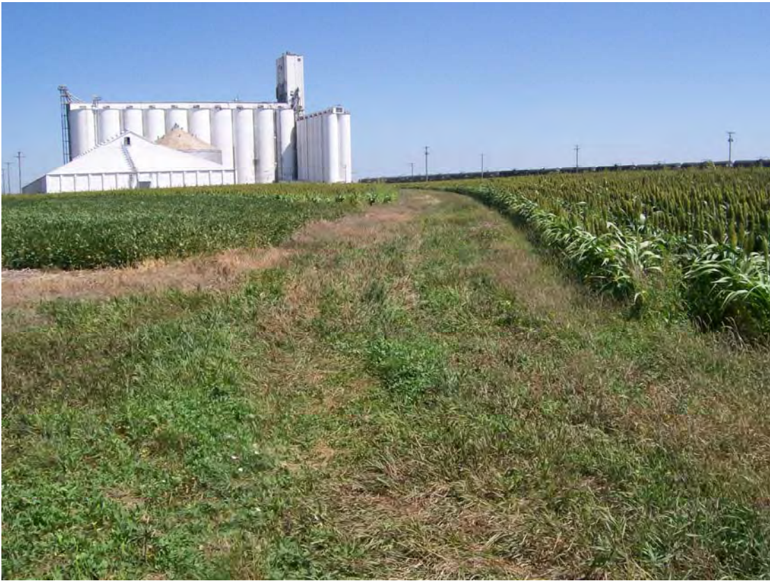
Looking northeast up the drainage ditch toward the Garvey Elevator
