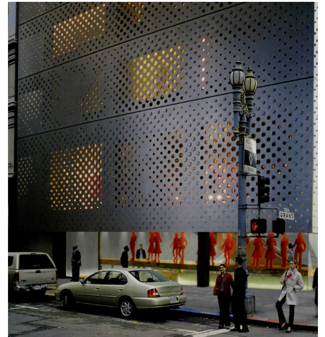
prada tower. office for metropolitan architecture. punctured sheets of steel. unlike the prior three buildings these examples push the boundaies of what is possible with a material like steel. not only do they push the boundaries but they also inspire those who come in contact with the buildings. anything from a facade of woven stainless steel strips to a sculpted facade of steel sheets is possible. even a material which is typically seen as stable and im- pervious can quickly be put into a state that chal- lenges that assumption.
