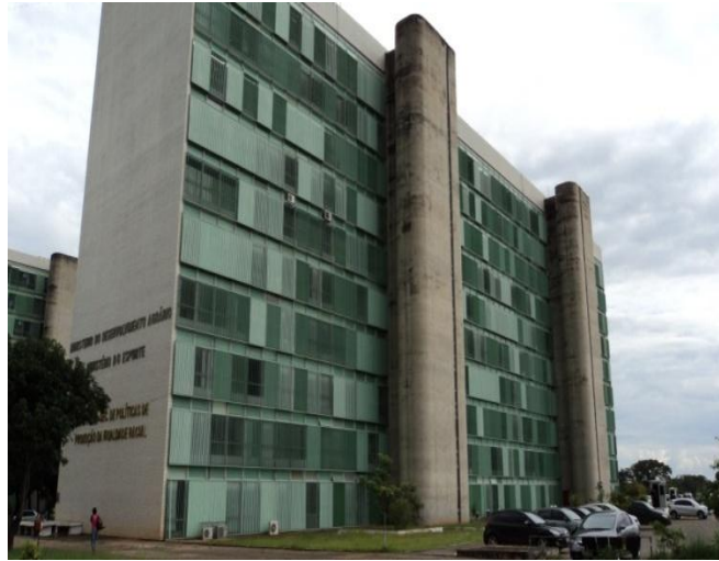
Figure 1 - Vertical blinds (louvers), control element in the west facade of Ministries in Brasilia, Distrito Federal (ARAÚJO, SIMÕES & SPOSTO, 2012)
