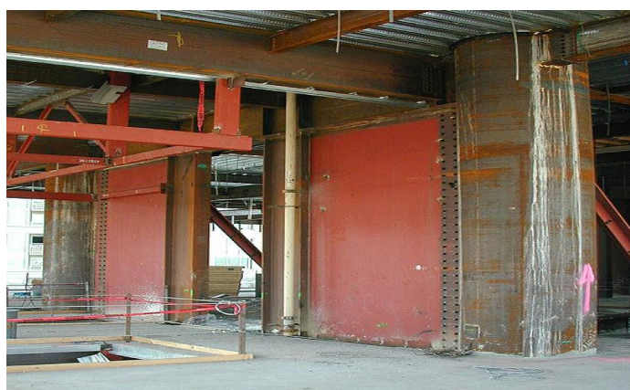
Figure 11: Coupled steel plate shear wall [9].
