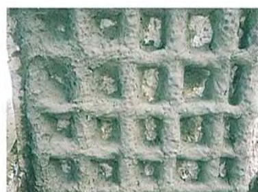
[J2モルタル施工]
