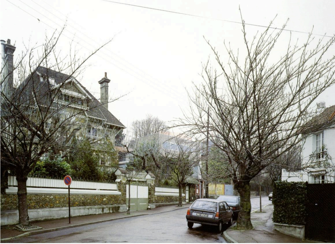
Photographs of built project
