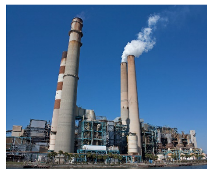
Figure 2-8 Fossil fuel power station
