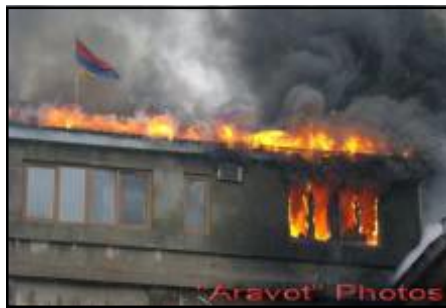
Fire gutted building housing the Armenian Ministry of Justice
